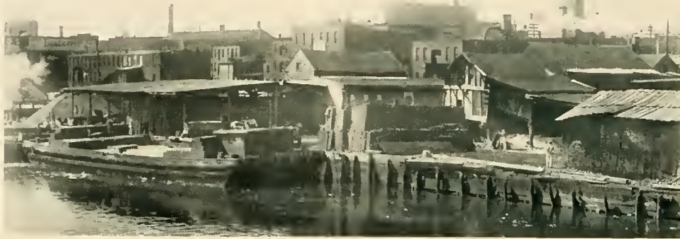
MAIN YARD, FOOT OF CENTRE STREET.
